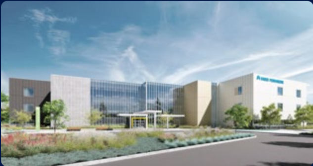
Modesto Medical Offices 2
