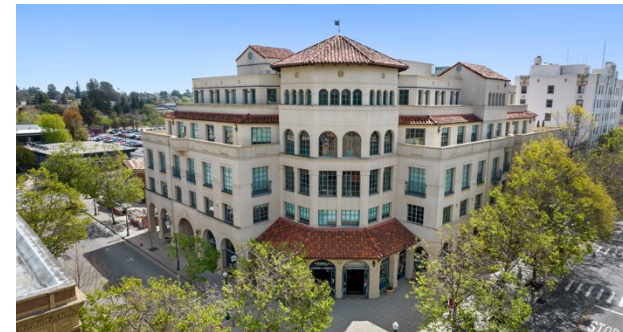
At the new Santa Cruz Medical Offices, members have access to family medicine, lab, mammography, ob-gyn, pediatric, pharmacy, and X-ray services.
